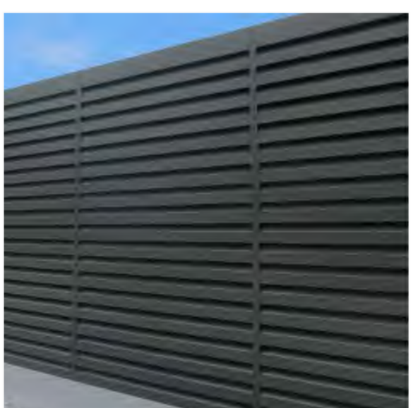
08 - Dark Grey acoustic louvers colour matched to zinc roof finish (05)
